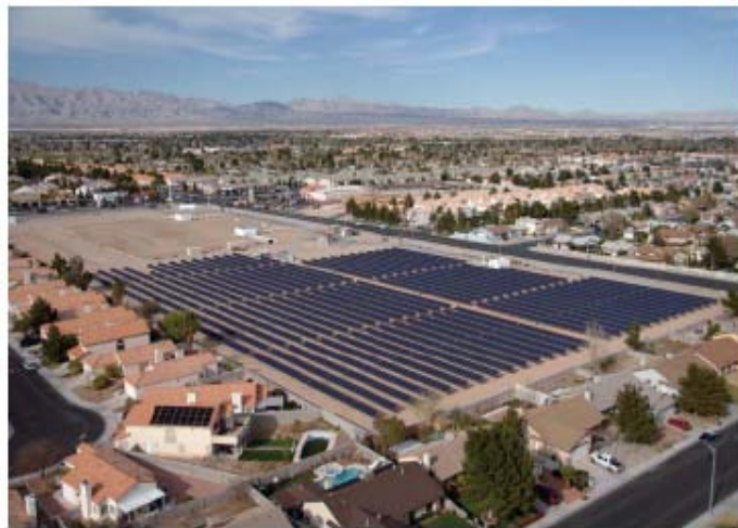
PowerTracker Ground System at the Ronzone Reservoir
